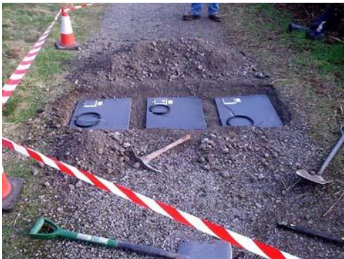
Pressure pads on unpaved path before being covered Photo Source: Scottish National Heritage
