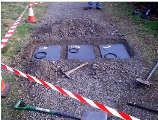
Pressure pads on unpaved path before being covered Photo Source: Scottish National Heritage
