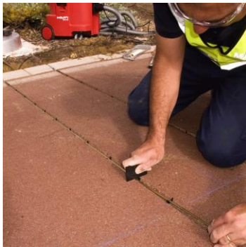
Installation of embedded piezoelectric strips Photo Source: Metrocount
