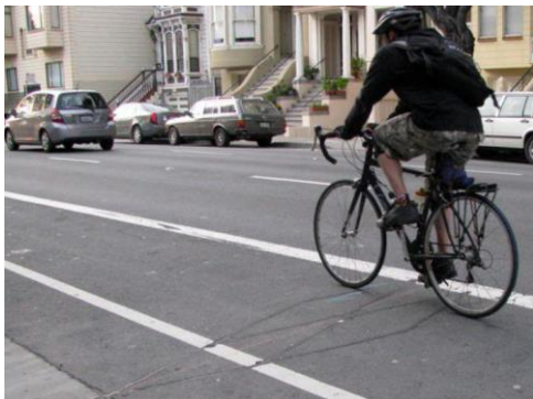
Embedded inductive loop detector in bike lane Photo Source: Ecocounter
